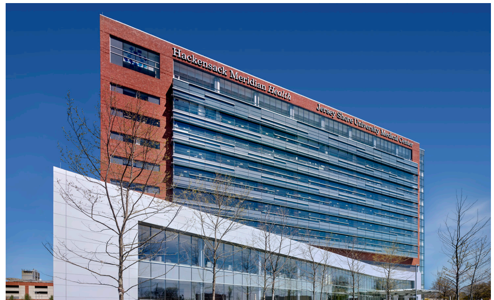
The design of the Healing Outpatient Experience Tower breaks the hospital stereotype by featuring expansive windows featuring Solarban ® 70 glass, which has a slight green tint that blends well with other green hues throughout the campus.
