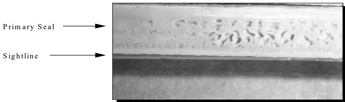
FIGURE-3 PRIMARY SEAL CAVITATION
