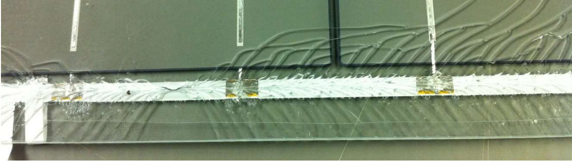
Photo 8. - Thermal Breakage at Frit
