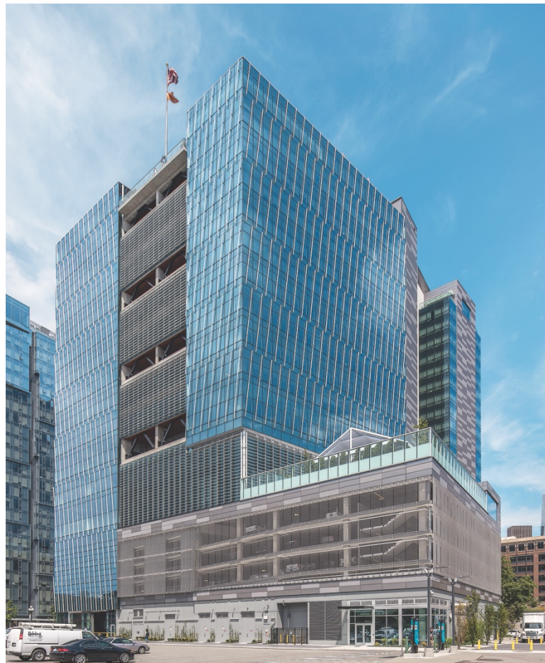
255 King, Seattle, WA, USA – Photos © Tom Kessler
